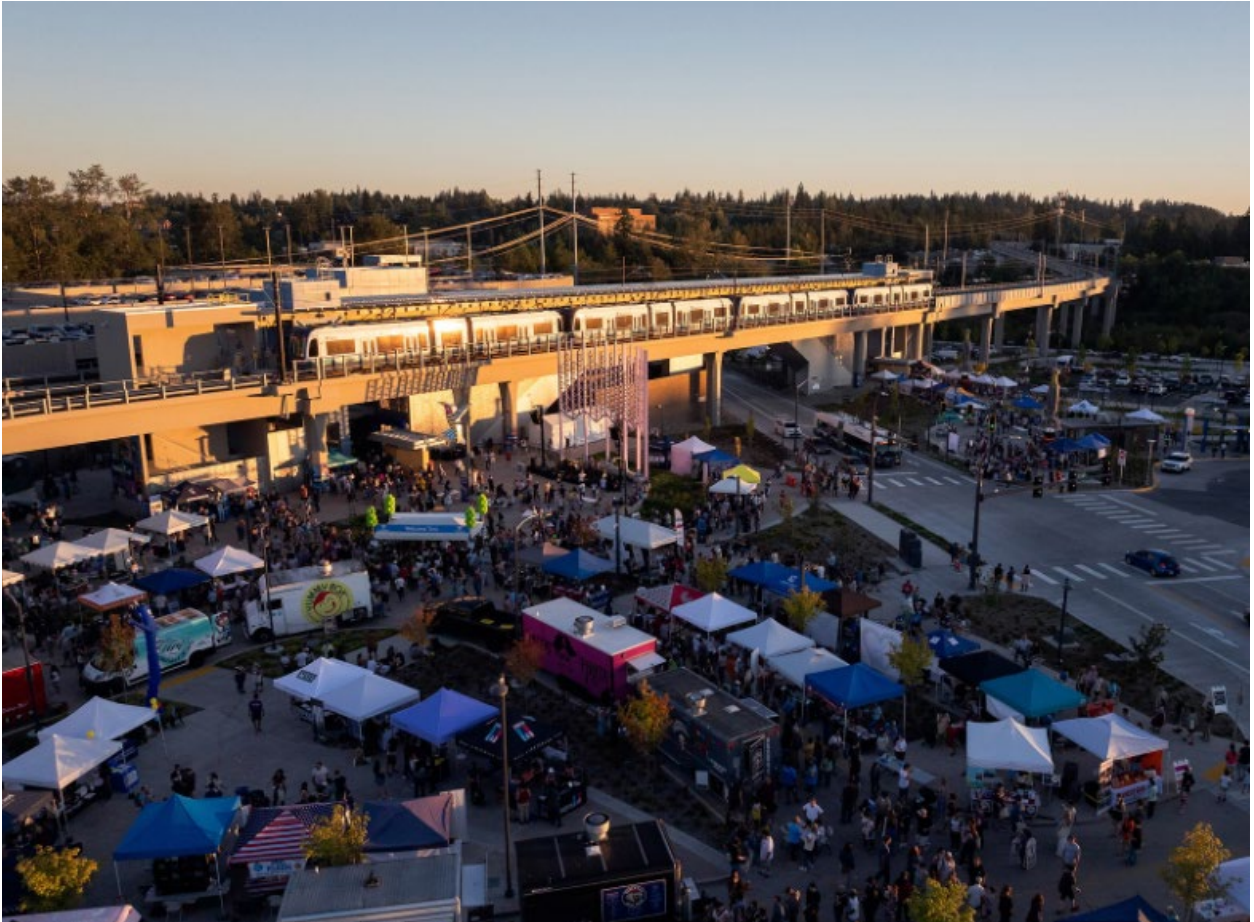
Opening Day Celebration at Lynnwood City Center Station, photo credit Sound Transit
